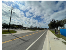
Newly paved road on Myrtle Ave between Booker High School and several industrial and manufacturing plants, 2023.
